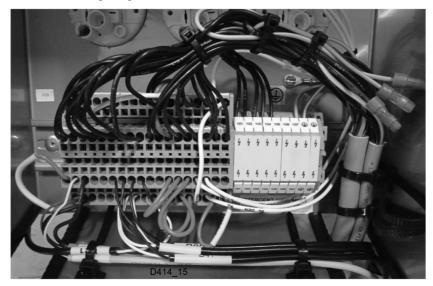
Check that all wiring has been connected. N.B.! Perform an additional check of the earth wiring.
