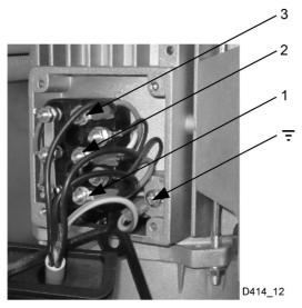
• Connect the wiring for the door switches to the terminals in accordance with the labelling.
